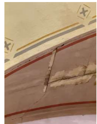
A closer look at the hole caused by the leak
