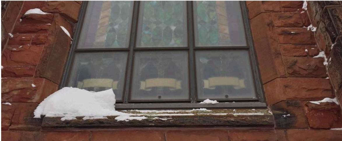
Stained glass windows were restored, repaired or replaced in 1997. 20 years of weather have taken their toll on some of the frames.
