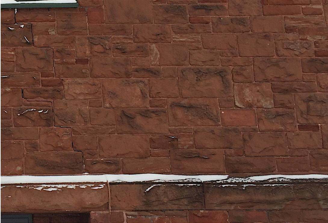
Mortar between the sandstone block deteriorates, causing the blocks to shift and leak. Both the back and front of the building had places with significant deterioration. A few places on the sides showed problems and repairs in the stones around the glass blocks were needed.
